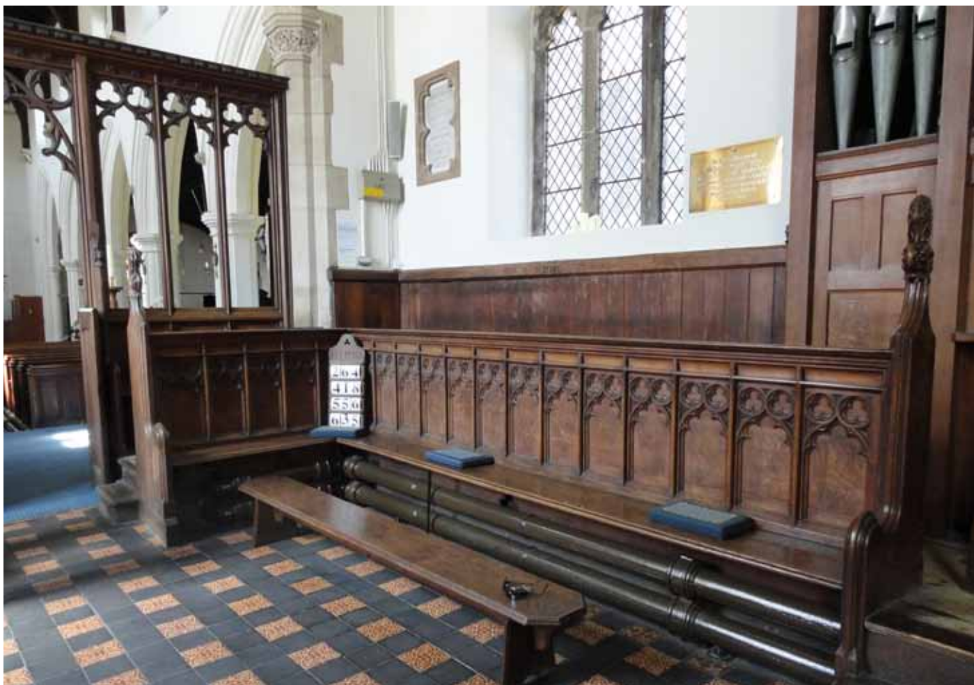
Below: North side of Quire; the organ and its 'chamber' are later additions, and I doubt very much if Pugin would have approved of them; nor possibly, of the heating pipes?
