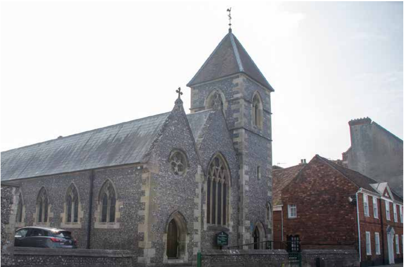
St Osmund's exterior. The north aisle was added in 1894 and was not part of Pugin's plans. Pugin's drawings are still held by the church. (John Elliott)
