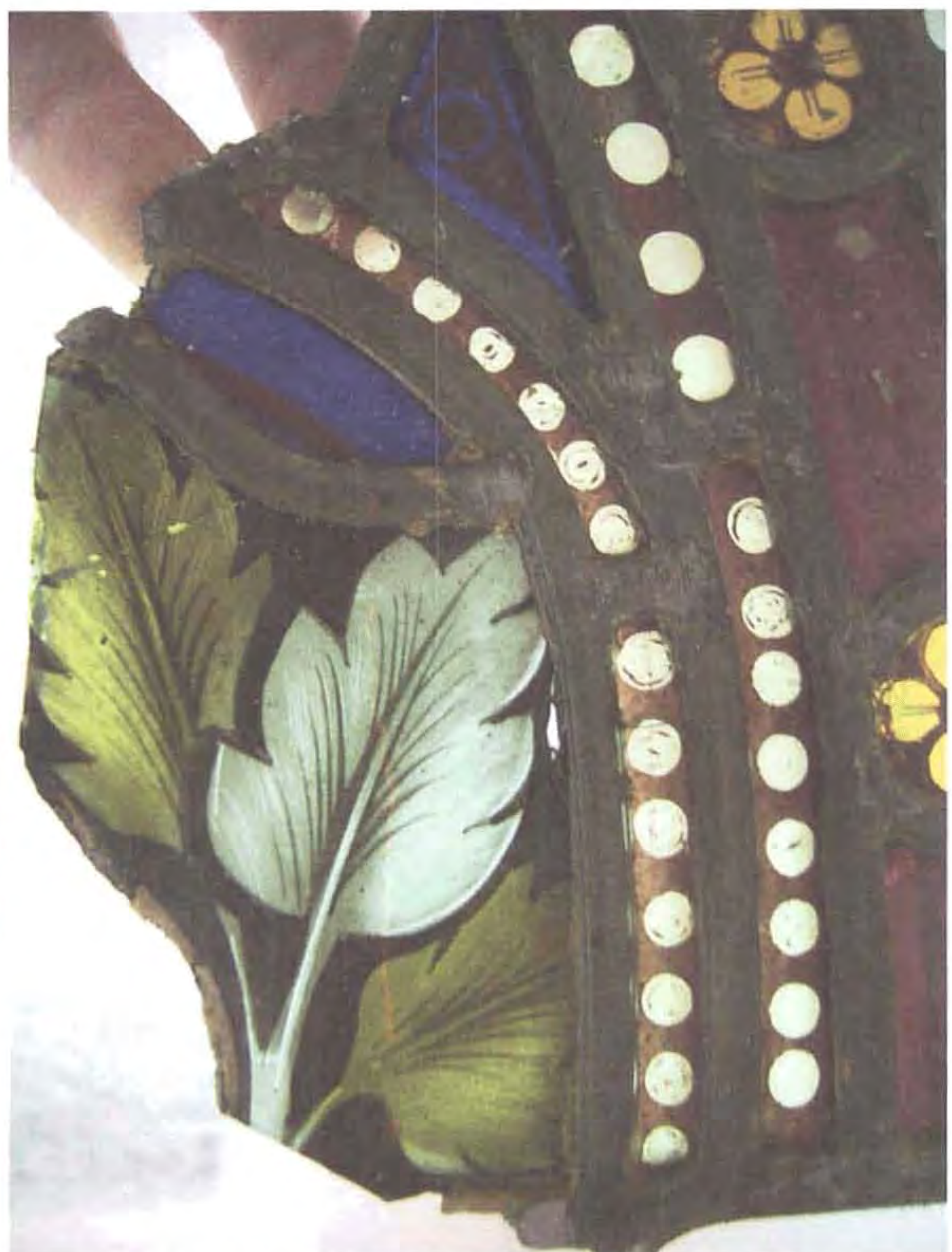
Figure 40: Poorly cut glass, its edge not completely covered by the lead calme
