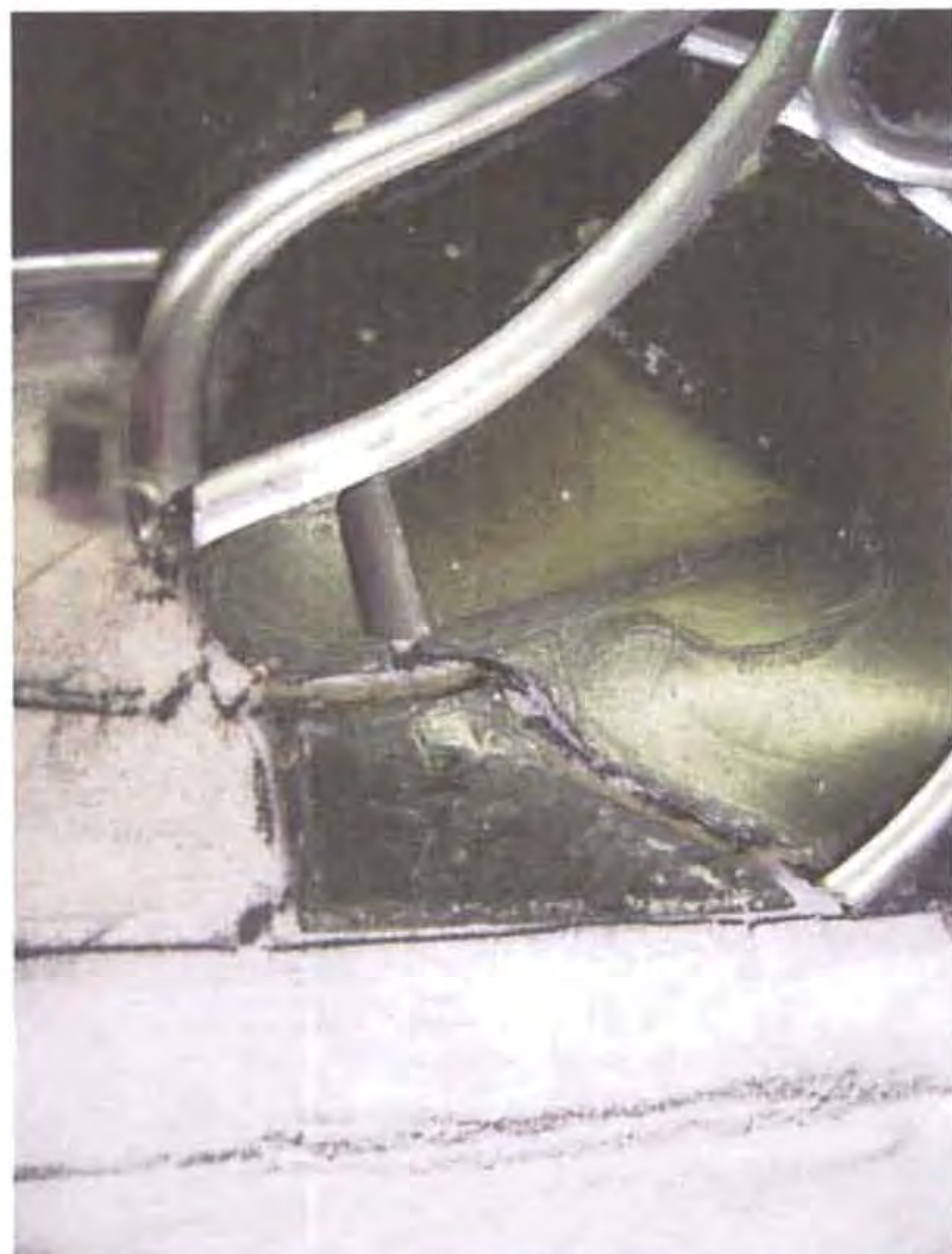
Figure 39: Ill-fitting adjacent pieces of glass
