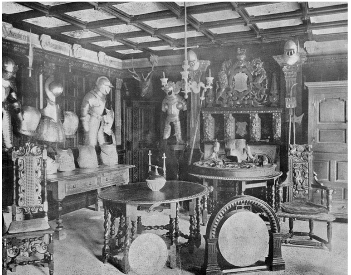
The Hall at St Chad's, Uppermill, from the 1920 auction catalogue. Image in the Public Domain.
