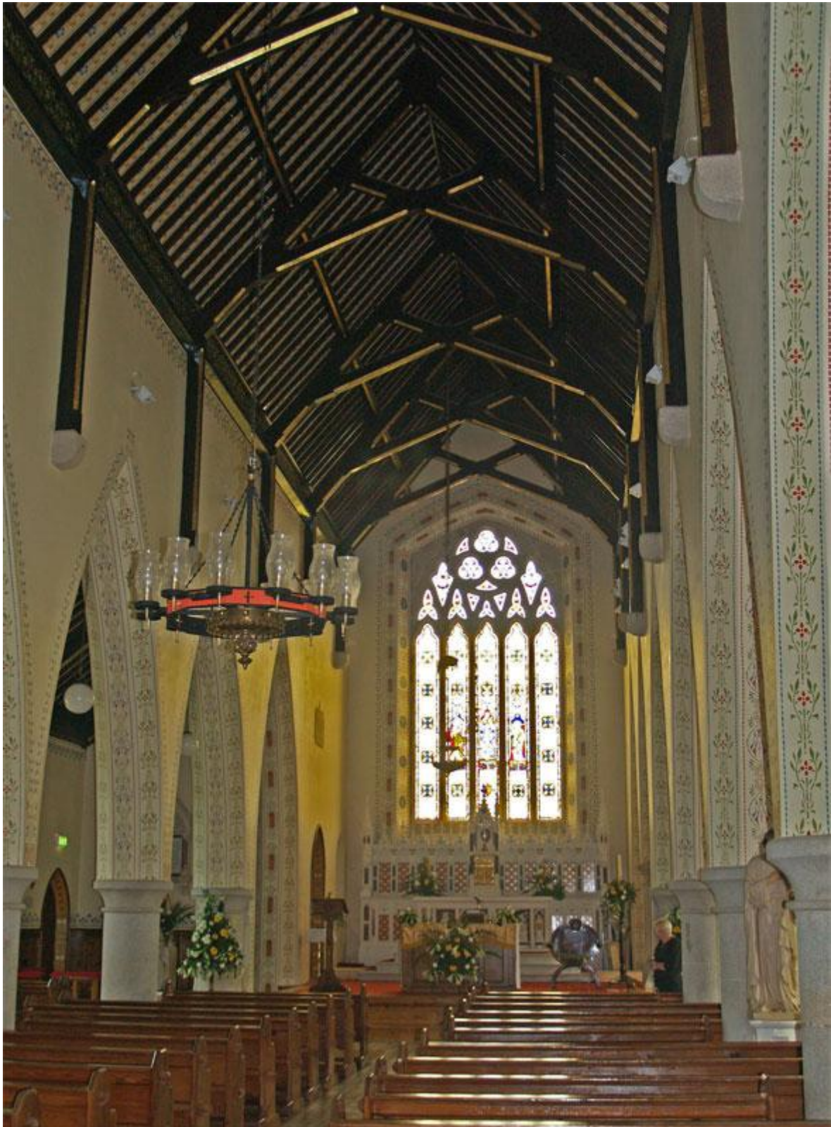
Nave roof trusses (Image: Brian Andrews)
