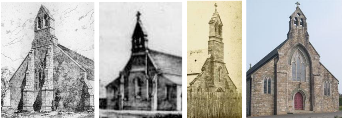
From the left: the Long Stanton, Cambridge, Ryde and Barntown facades
