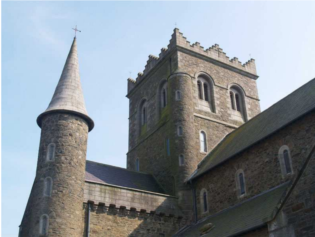
Corbelled walkway on the north transept west wall giving access from the round tower stairwell to the clasping circular stairwell on the crossing tower north west corner (Image: Brian Andrews)
