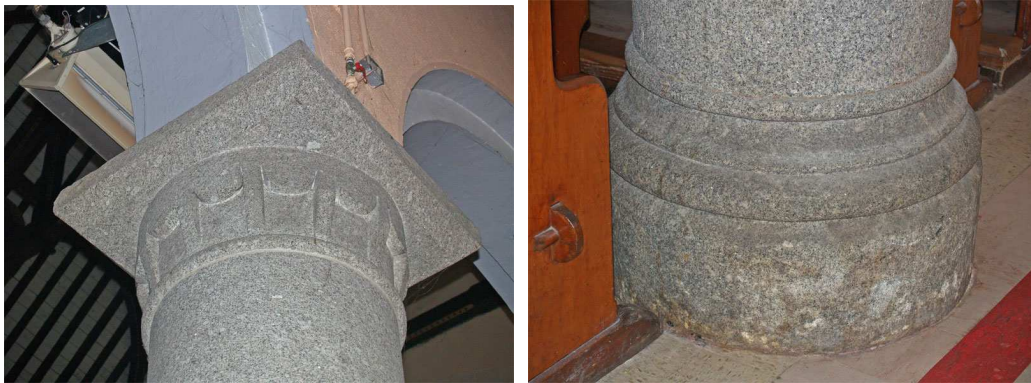
Nave arcade capital and base (Images: Brian Andrews)
