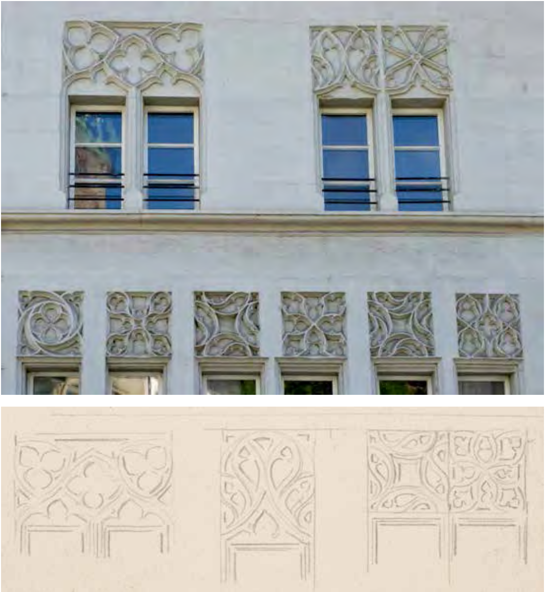
Fig.6 (a) Tracery of one house at the rue de la Neuveville in Fribourg. Photo Oscar Pugin . Fig.6 (b), Pugin's study of the traceries. © Victoria & Albert Museum, London
