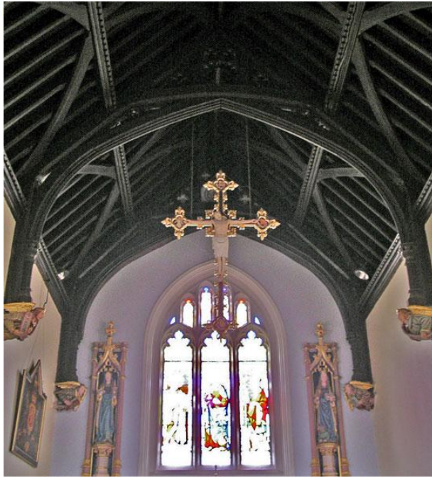
Two levels of windbracing in the original nave and chancel of St John's Hospital Chapel, Alton (Image: Nicholas Callinan)
