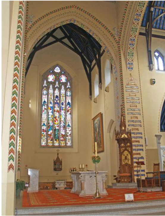
A view into the north transept of St Aidan's Cathedral showing the arch-braced roof (Image: Brian Andrews)
