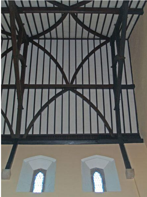
Above, the Tagoat nave roof; below, a view along the nave looking east, showing the wind bracing in the transepts (Images: Brian Andrews)
