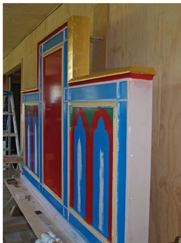
Above, the two-dimensional mock-up; below, the reredos with some base colours & gilding (Images: Brian Andrews)
