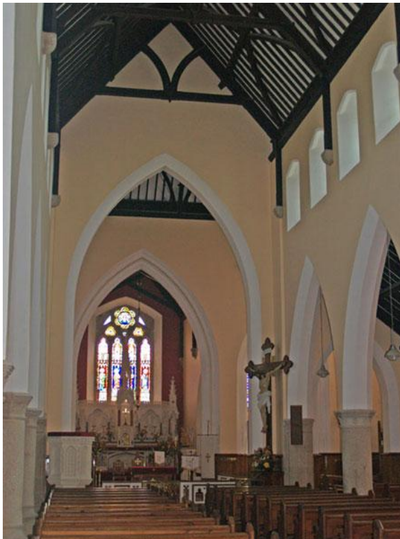
Above, the Tagoat nave roof; below, a view along the nave looking east, showing the wind bracing in the transepts (Images: Brian Andrews)
