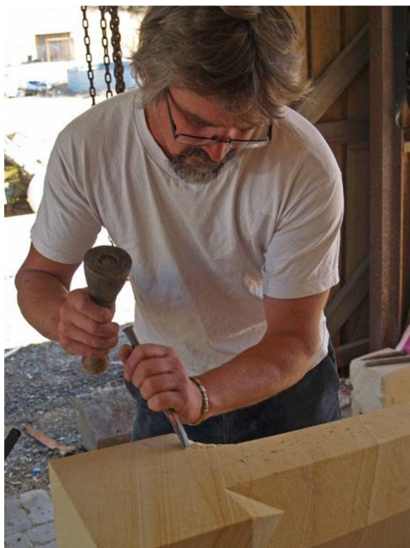
Above and below: Edrei Stanton carving the base of the shaft for the Richmond churchyard cross (Images: Brian Andrews)
