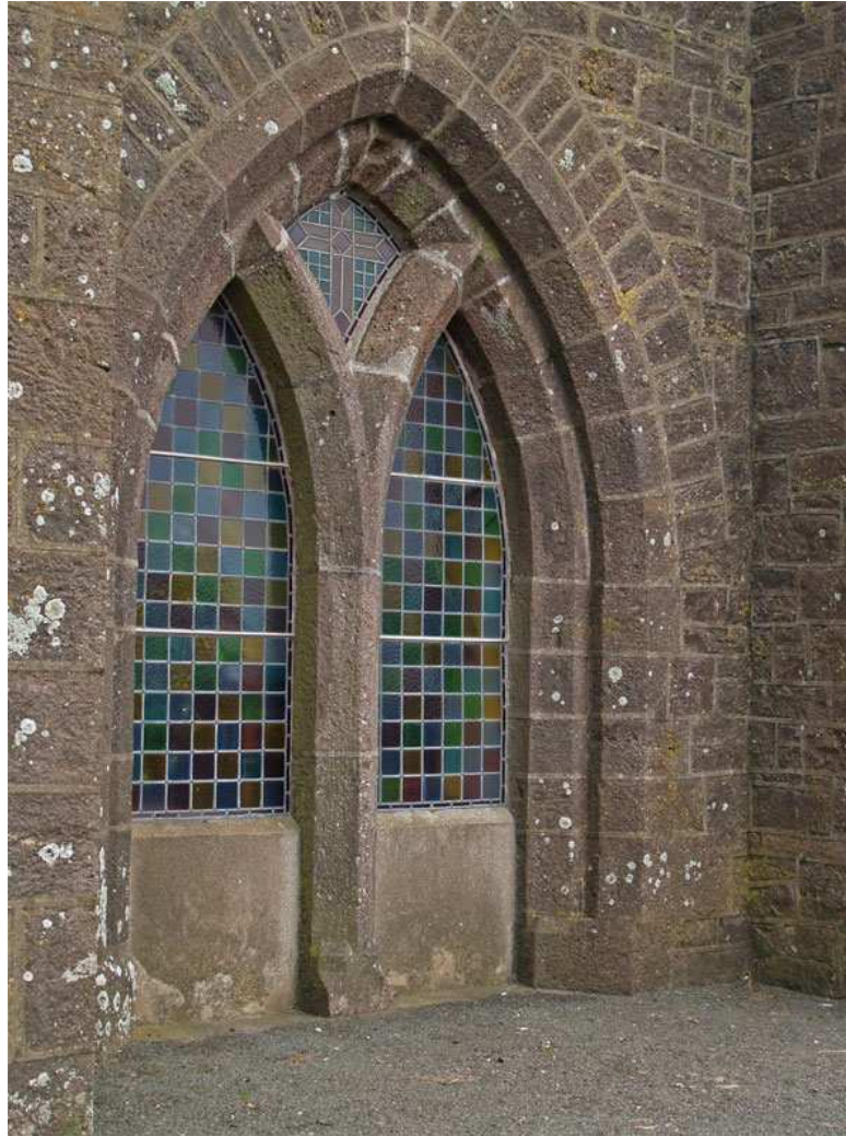
Blocked-up west door in tower (Image: Brian Andrews)
